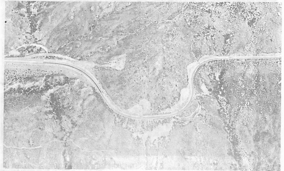
TREACHEROUS VIEJAS GRADE SHOULD BE COMPLETED. PHOTO BY AL HOWE.
